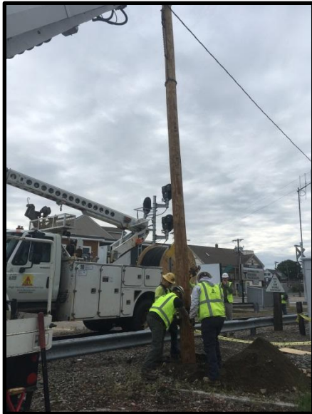
Wood Pole Installation
