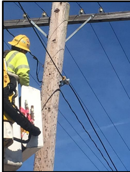
Overhead F.O. Installation
