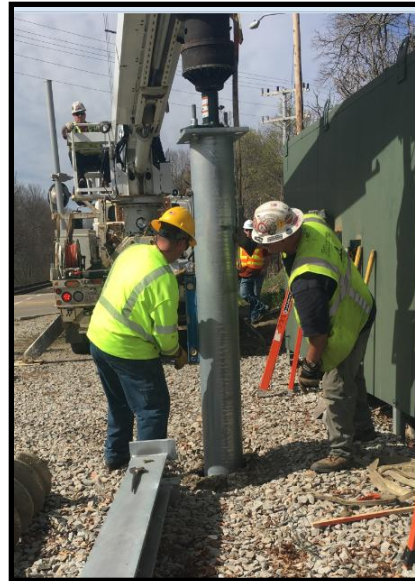
Antenna Base Installation
