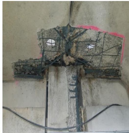
Concrete Repair Preparation
