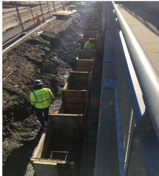
CR Walkway Canopy Footings – Rebar and Forms
