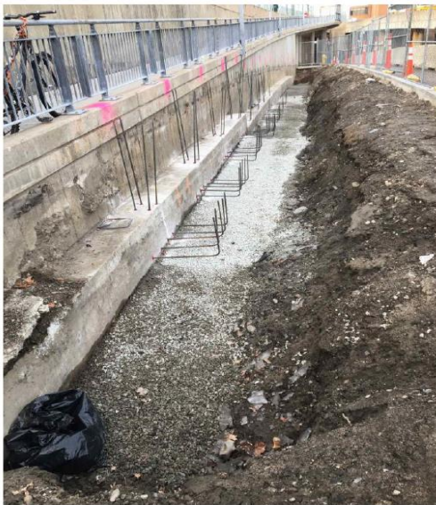
CR Walkway Canopy Footings – Rebar and Forms
