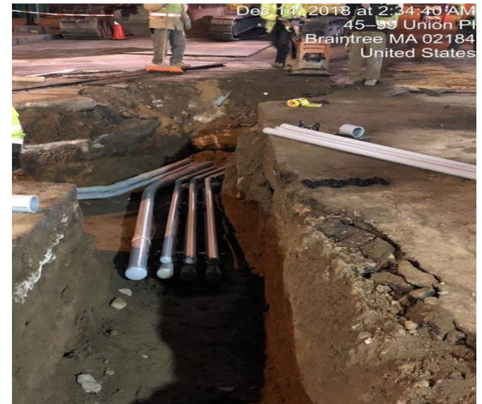
Conduit Installation at Busway
