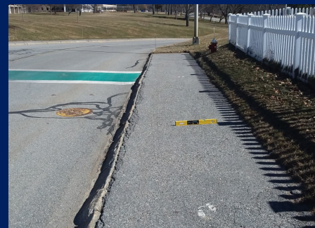
Missing curb ramp
