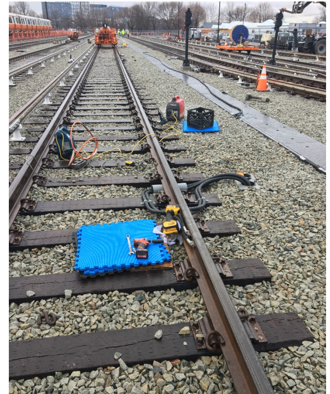
Completed Track Bonding T35 North
