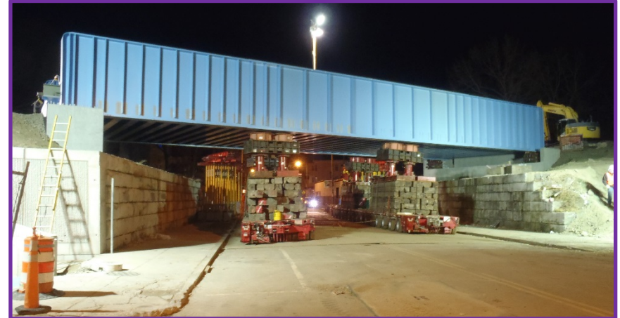
Bridge Lowered to Precast Bridge Seats
