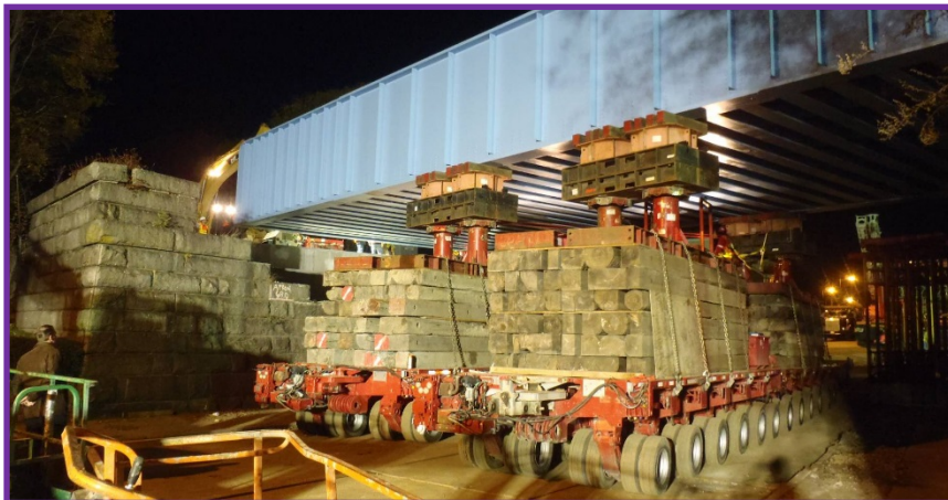
Saturday Night – Bridge moved into place
