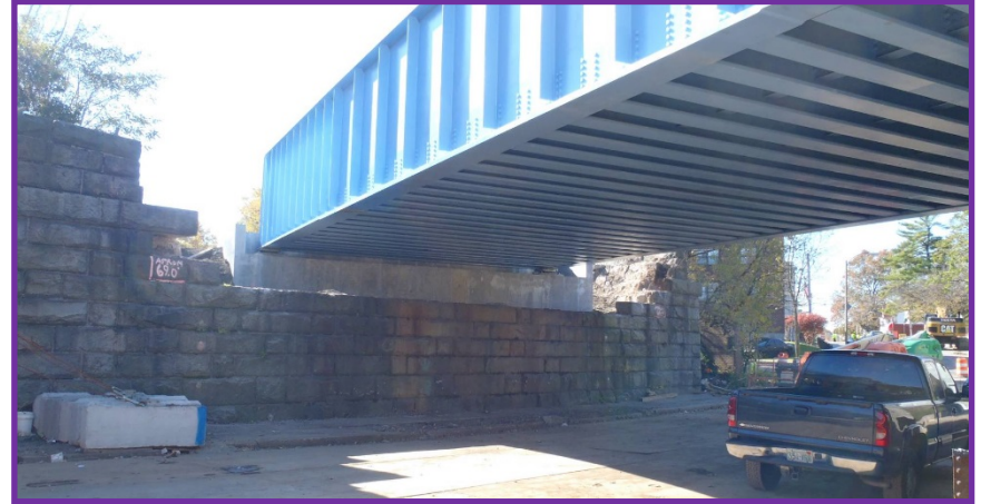
Sunday – Bridge in Place
