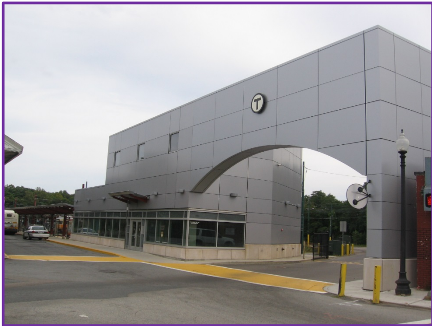
New Station Building
