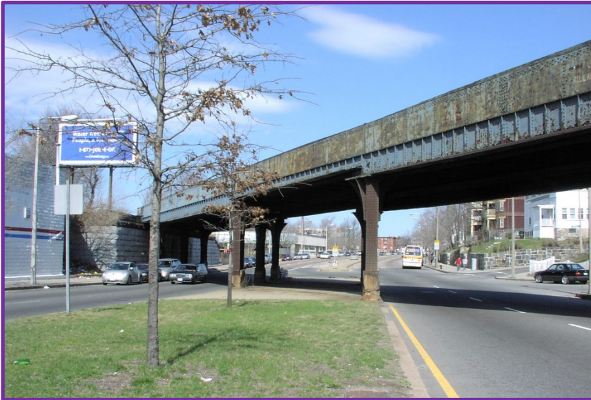
Original Columbia Road Bridge
