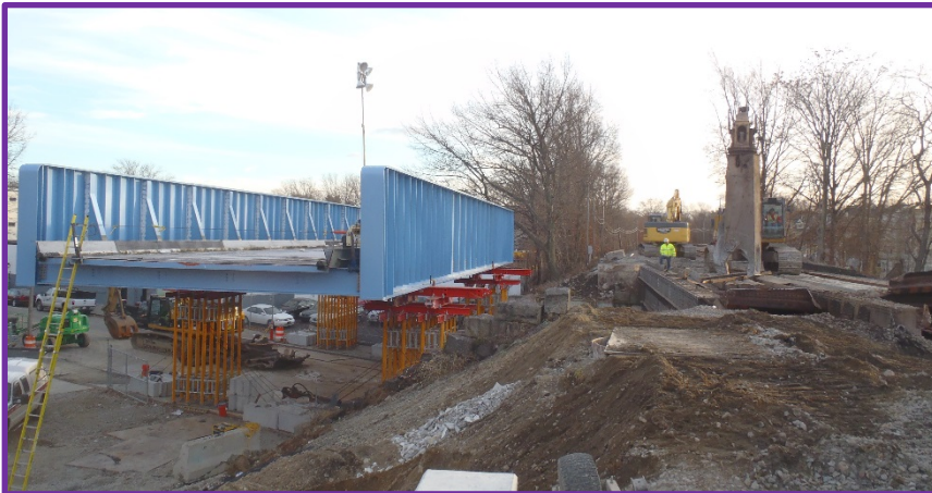
Single Weekend Demo and Installation
