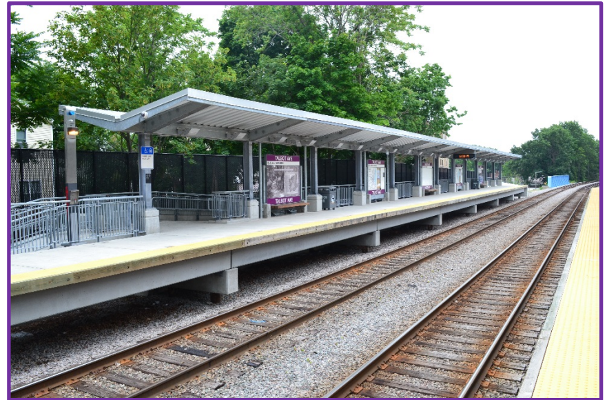
Inbound Platform and Canopy
