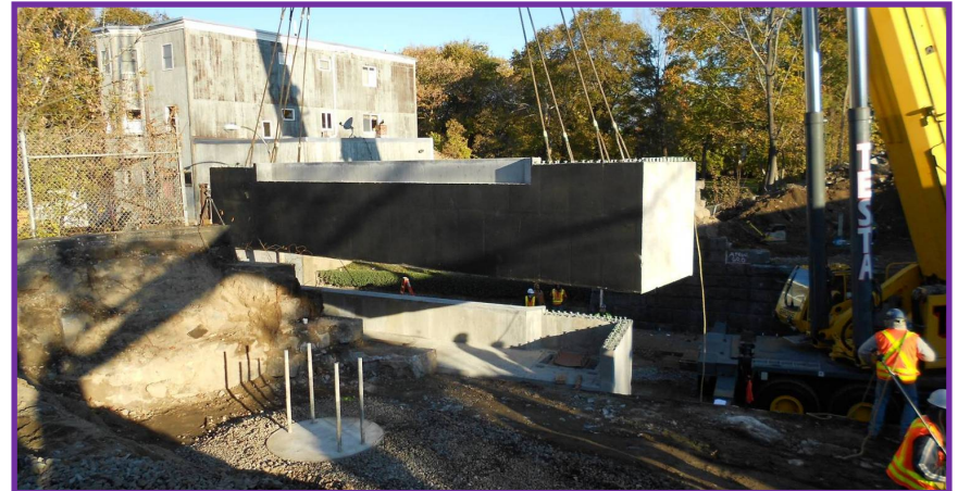
Saturday Morning – Precast Bridge Seats
