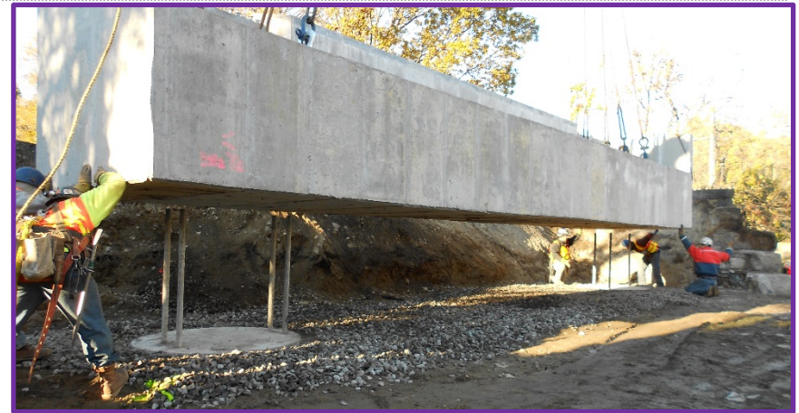
Precast Bridge Seat on Drilled Shafts
