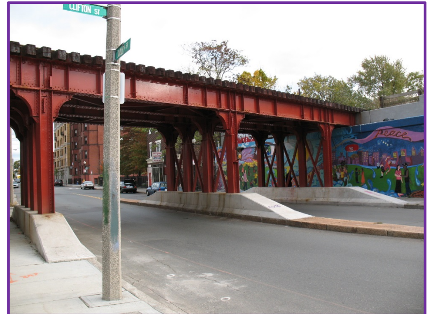
Repaired Dudley Street Bridge
