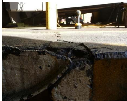
Figure 13 - Quincy Garage Pit Structure
