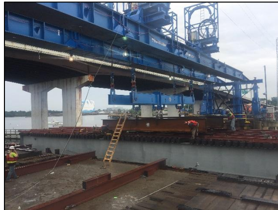
New bridge span in place
