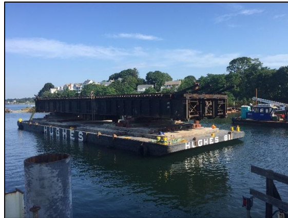
Old bridge span removed and on barge
