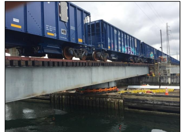
Test train running on bridge
