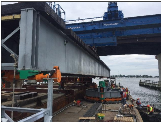
Moving the new bridge span into place
