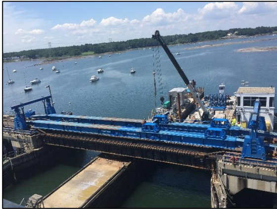
Preparing to remove the existing span
