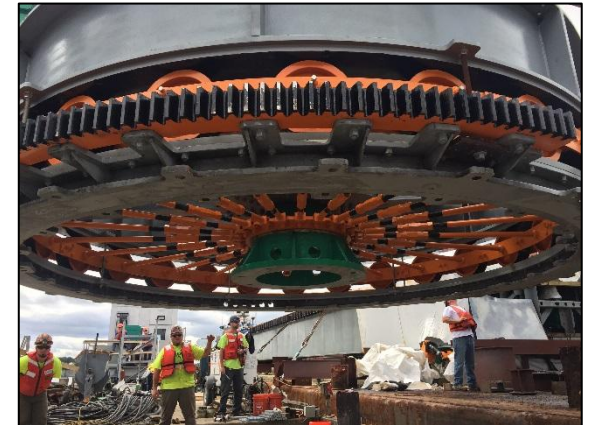
Drum girder and center pivot being lowered into place
