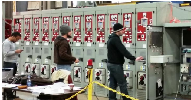
New Metal Enclosed DC Switchgear being Factory Tested
