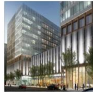
Assembly Row- Assembly Station, Somerville
