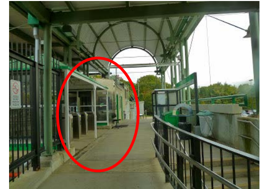
Riverside Station fare gates. Photo by @milesonthembta
