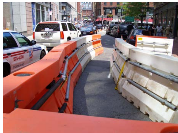
Safety barriers along both sides of temporary pedestrian access route
