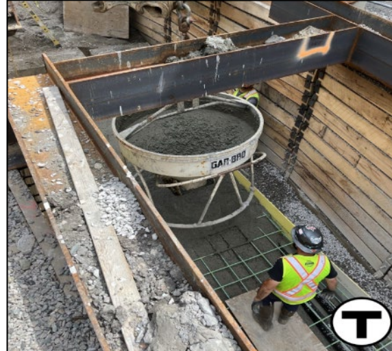
Duct Bank – Concrete Placement
