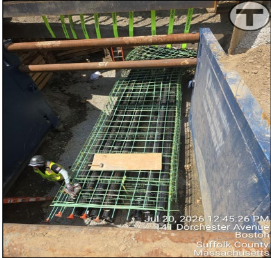
Duct Bank-Conduit and Reinforcing Steel Installation
