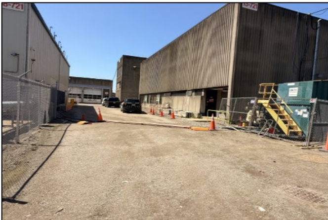
Completed Work Area – Restored to MBTA Operations
