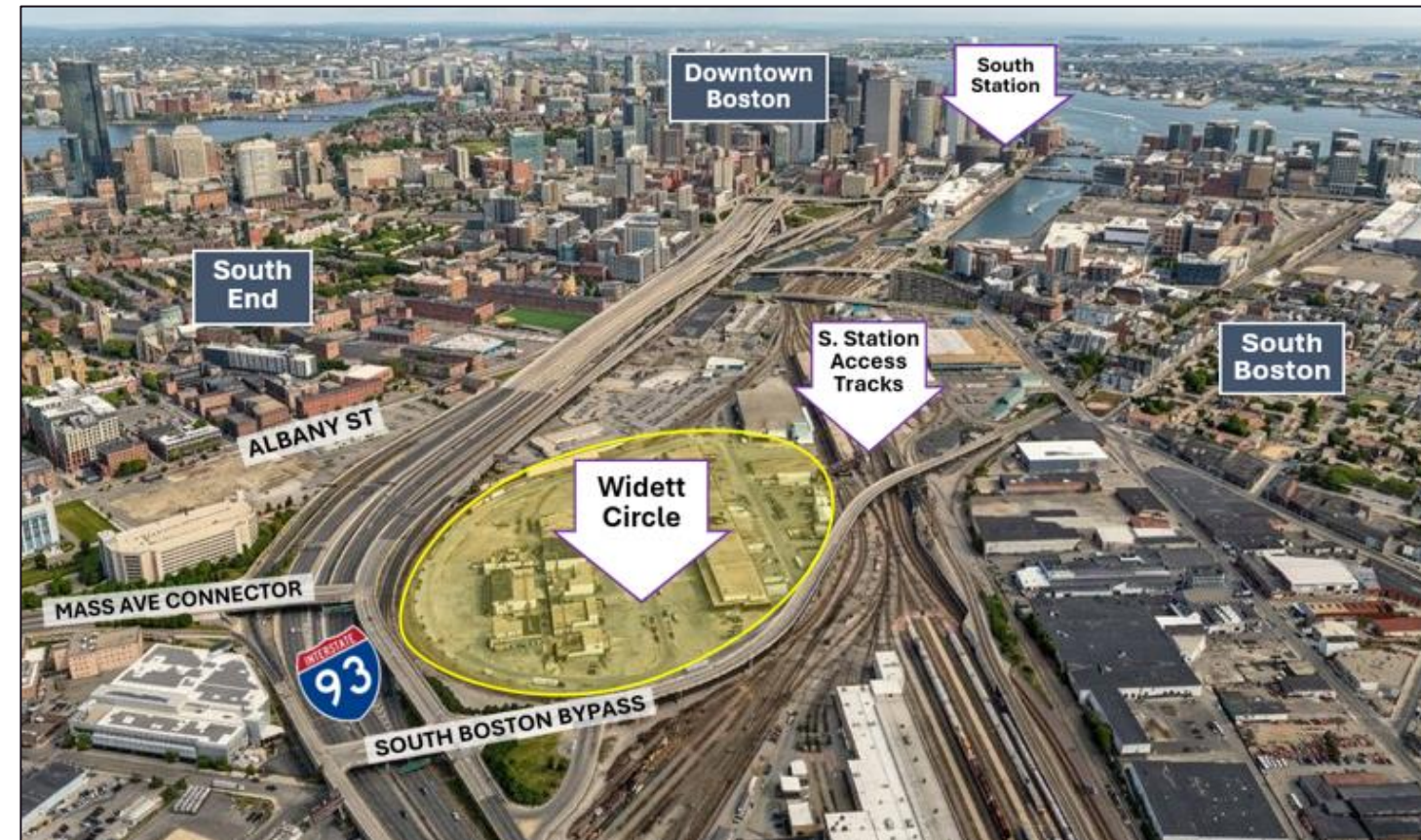
Aerial of Widett Circle site.
