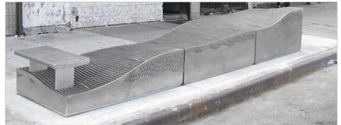
Figure 21: Vent shaft covers such as the one pictured to the right from the Metropolitan Transportation Authority (MTA) in New York City, can both passively protect vent shafts from flooding while also providing public benefits, such as seating and placemaking. The bench pictured is one option to consider while piloting passive mitigation strategies for vent shafts.
