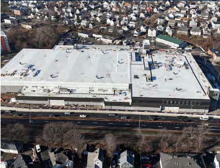
Jan. 2026 aerial view of new Quincy facility
