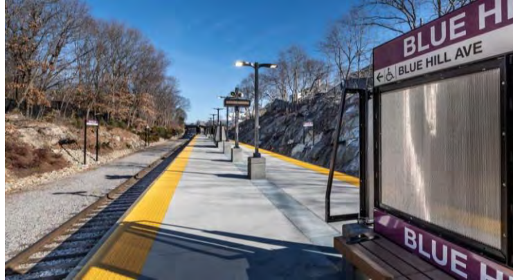
Blue Hill Ave station and track on Fairmount Line
