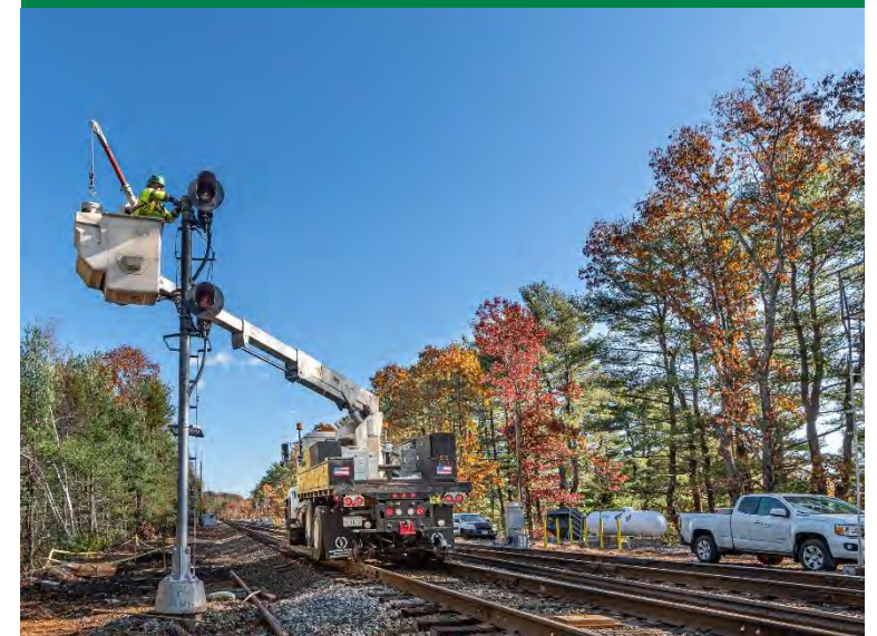
Signal work near Kendal Green Station
