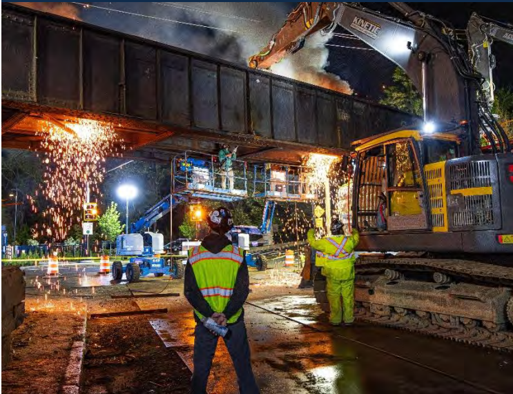
Haverhill Line bridge replacement
