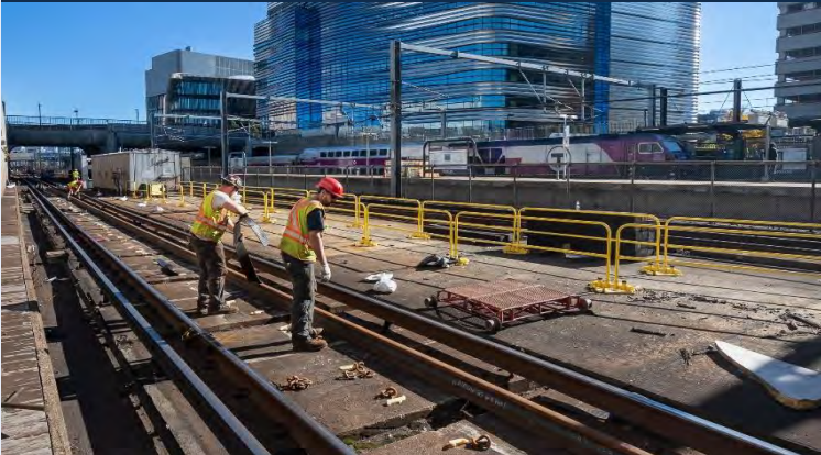
Orange Line track repairs near Ruggles Station
