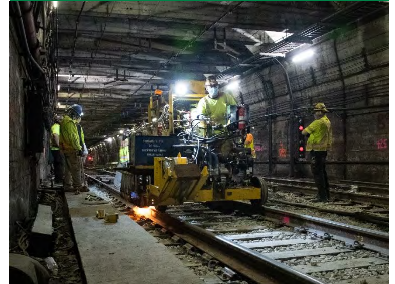
Trackwork near Airport Station on the Blue Line
