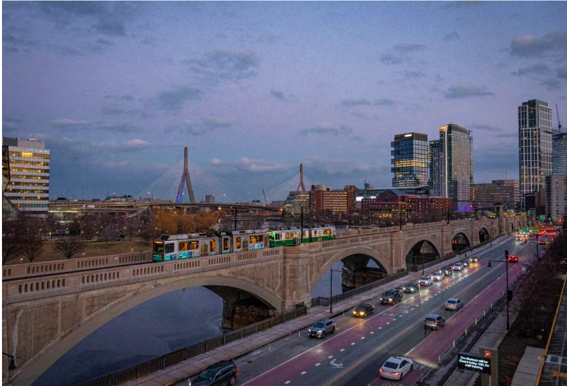
Green Line train passes over Lechmere Viaduct
