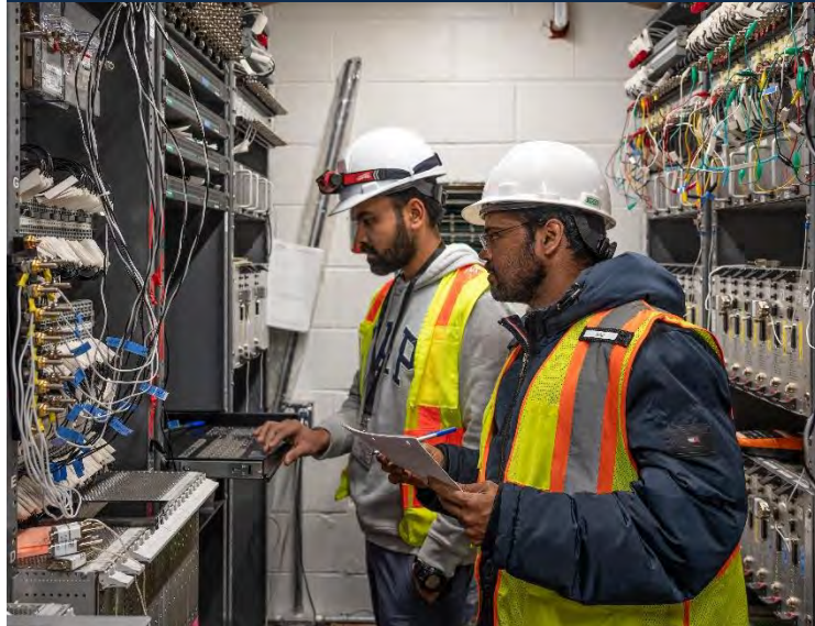
Staff working on Red Line signals at Quincy Center
