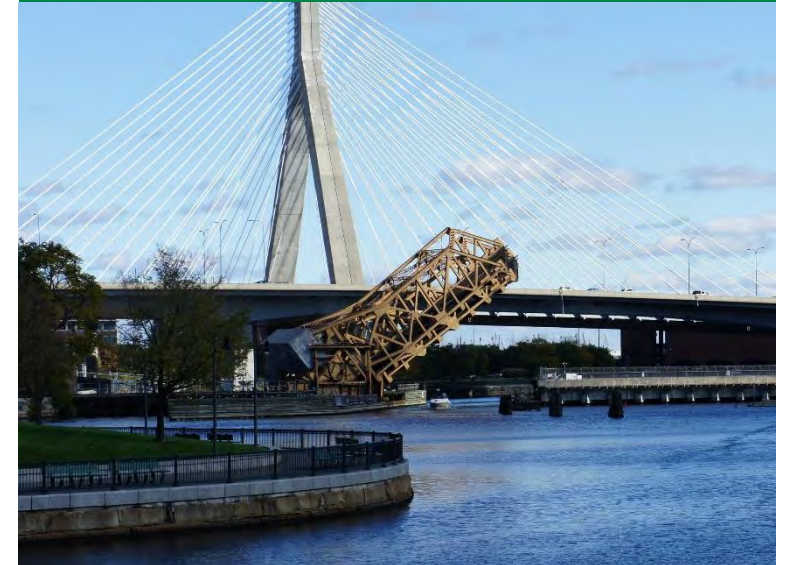
Existing North Station Draw 1 Bridge, built in 1931
