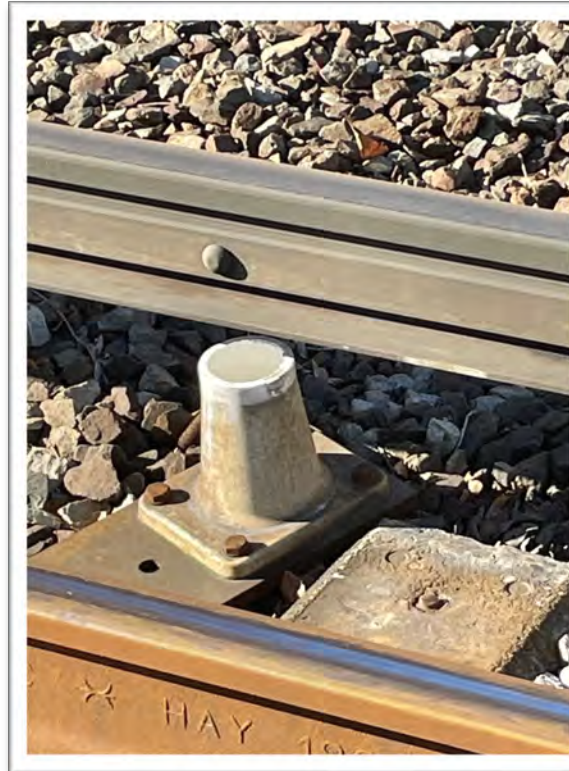
Broken rail insulator south of JFK/UMass observed in early December 2025.
