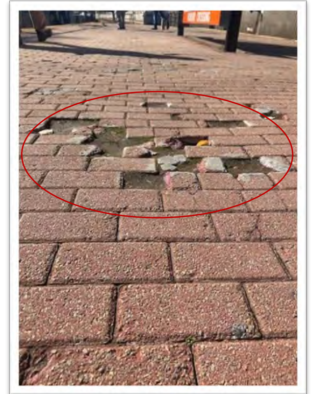
Tripping hazard (missing and loose bricks) at Roxbury Crossing.
