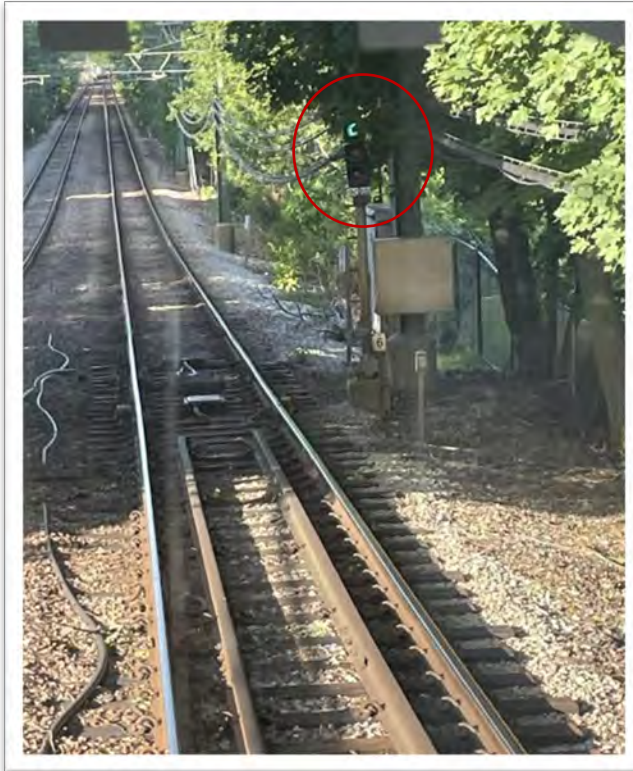
Vegetation obstructing signal visibility between Revere Beach and Beachmont.
