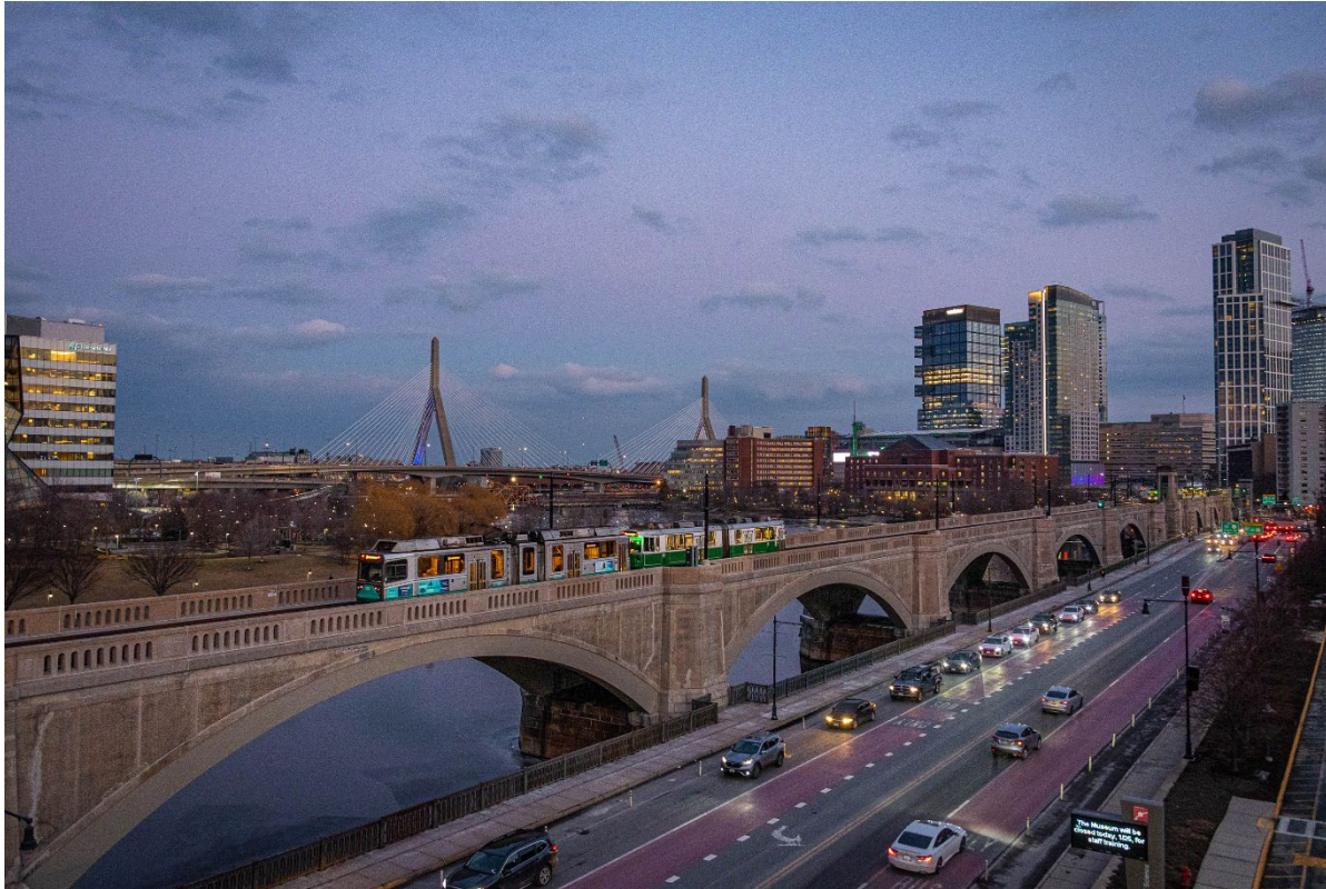
Green Line train passes over Lechmere Viaduct
