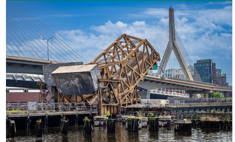
Existing North Station Draw 1 Bridge, built in 1931
