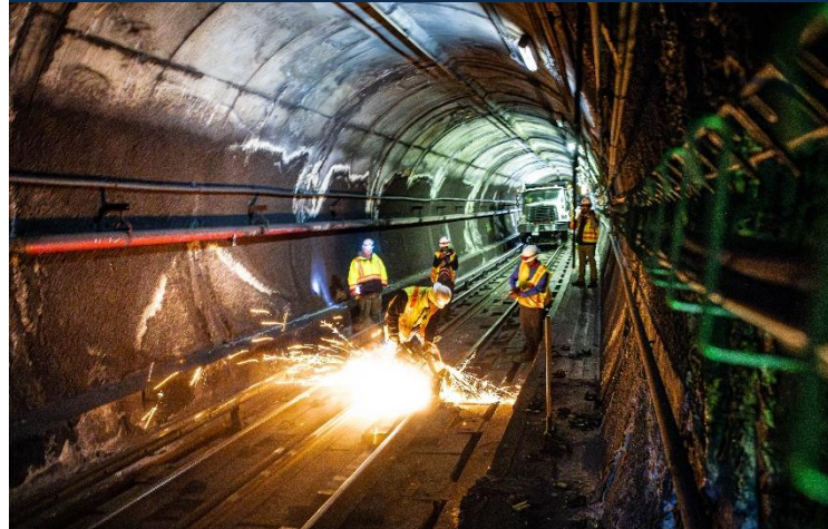
Red Line track work between Alewife and Porter Stations
