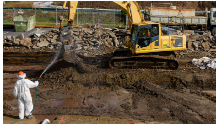
Example soil excavation
