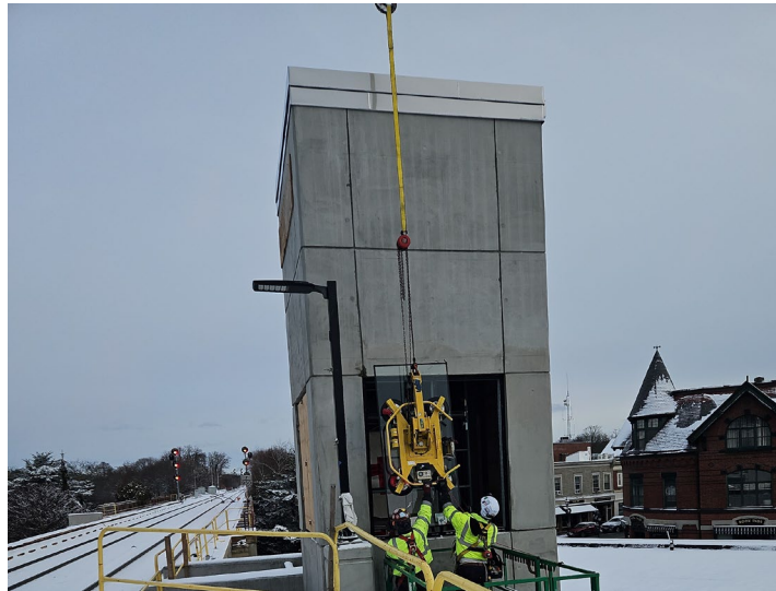
Window Installation, North Elevator
