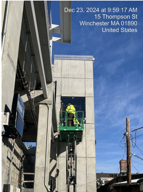
North Elevator Shaft Construction
