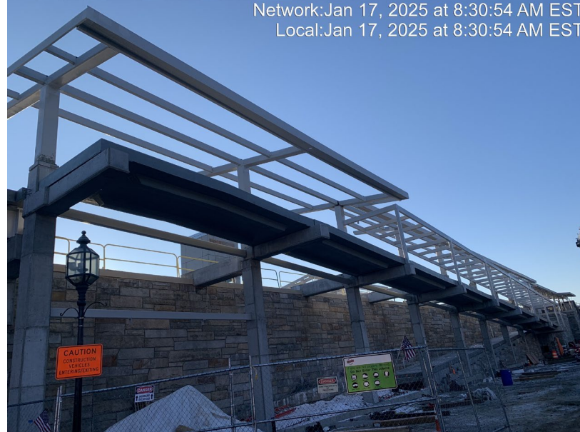
Inbound Platform Ramp Construction
