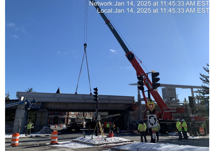
Platform Beam Placement over Quill Rotary
