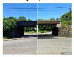
We're replacing the South Elm bridge which carries the Haverhill Line over South Elm Street between the Bradford and Haverhill stations. The current bridge was built in 1906, and replacement is necessary to extend its service life and bring it into a State of Good Repair.
