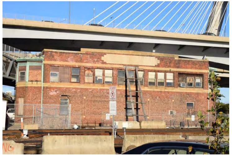
2. Existing Signal Tower A facing east from MBTA ROW.
