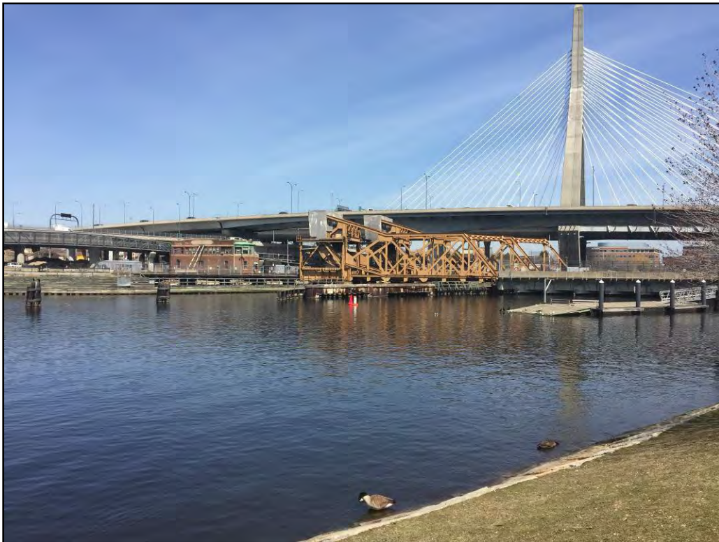
Figure 3. Overview of the project area from Nashua Street Park, Boston, looking northeast.
