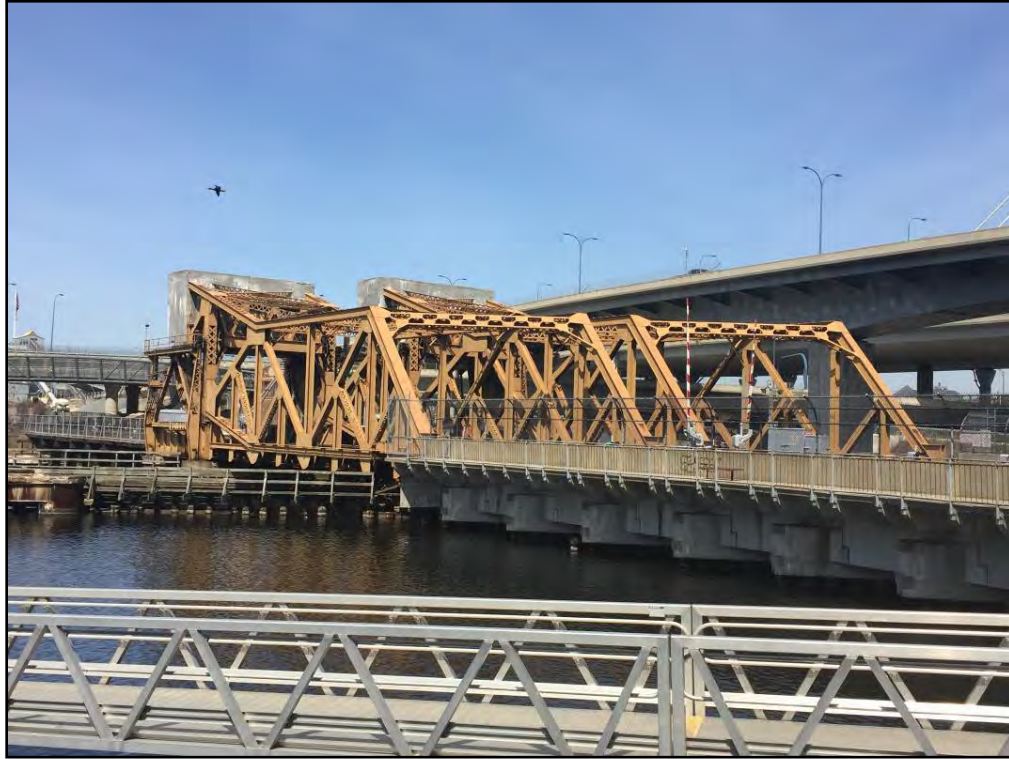
Figure 8. Draw 1 Bridges and south concrete pier approach span, looking northeast.
