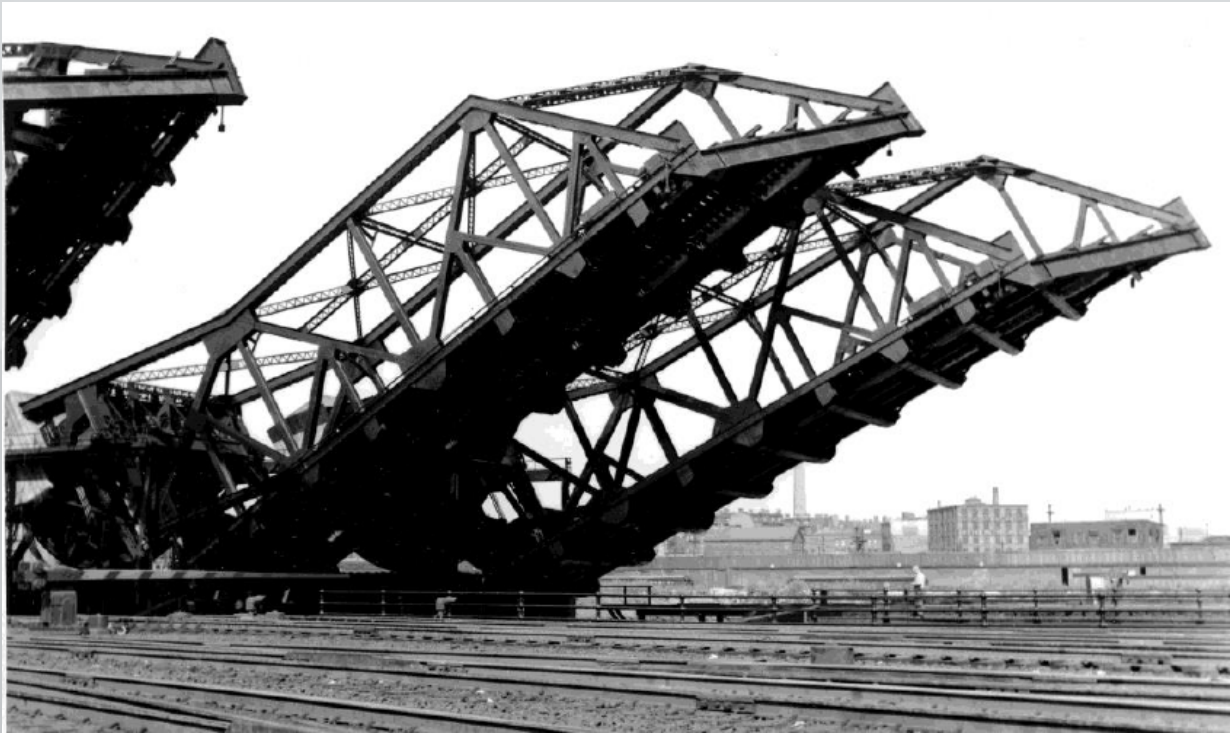
Draw 1, Spans 1 and 2, Boston Terminal. September 29, 1946
