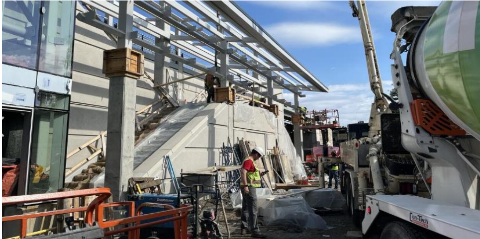
P0179 Winchester Center Station
