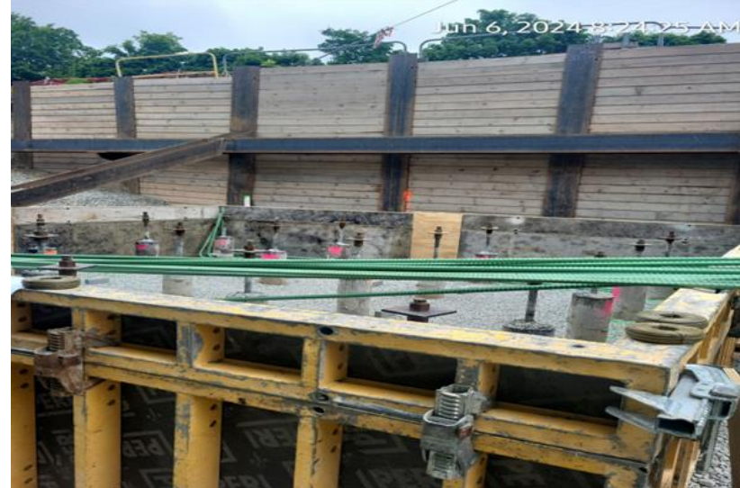
P0679 Codman Yard Expansion and Improvements
