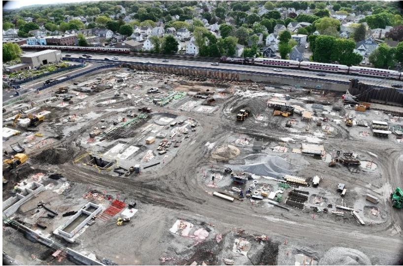
P0671a Quincy Bus Maintenance Facility Modernization
