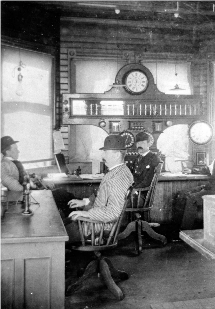
Old Tower A Control Room, 1884
