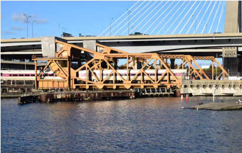
1. Facing east from existing Draw One Bridge.
