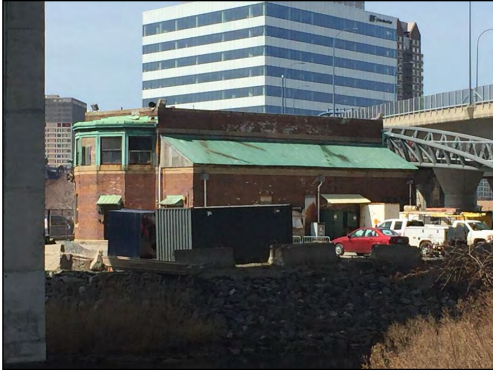
Figure 12. Signal Tower A, looking west at the east (rear) elevation.
