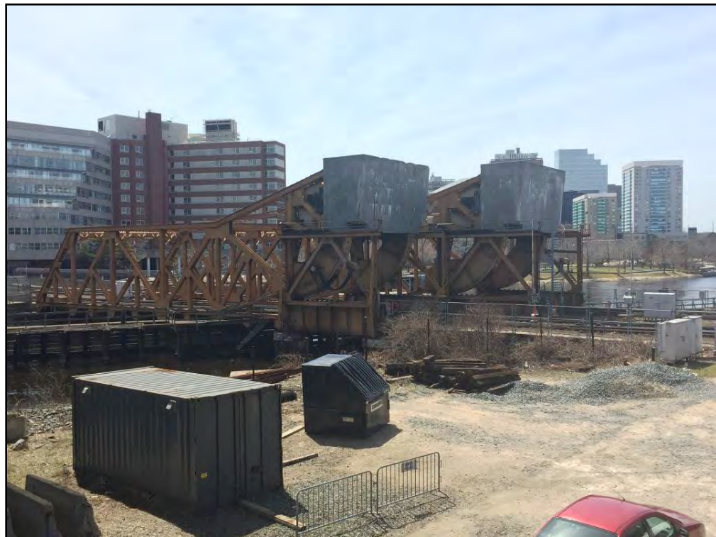
Figure 9. Draw 1 Bridges, looking southwest.
