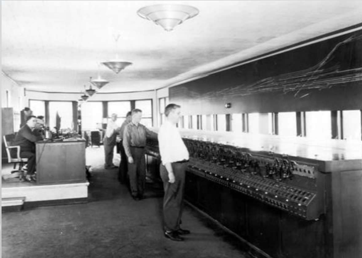
Interior of Signal Tower A control room. Date unknown
