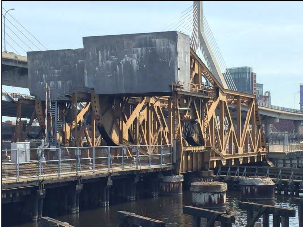
Figure 7. Draw 1 Bridges and north timber pile approach span, looking southeast.
