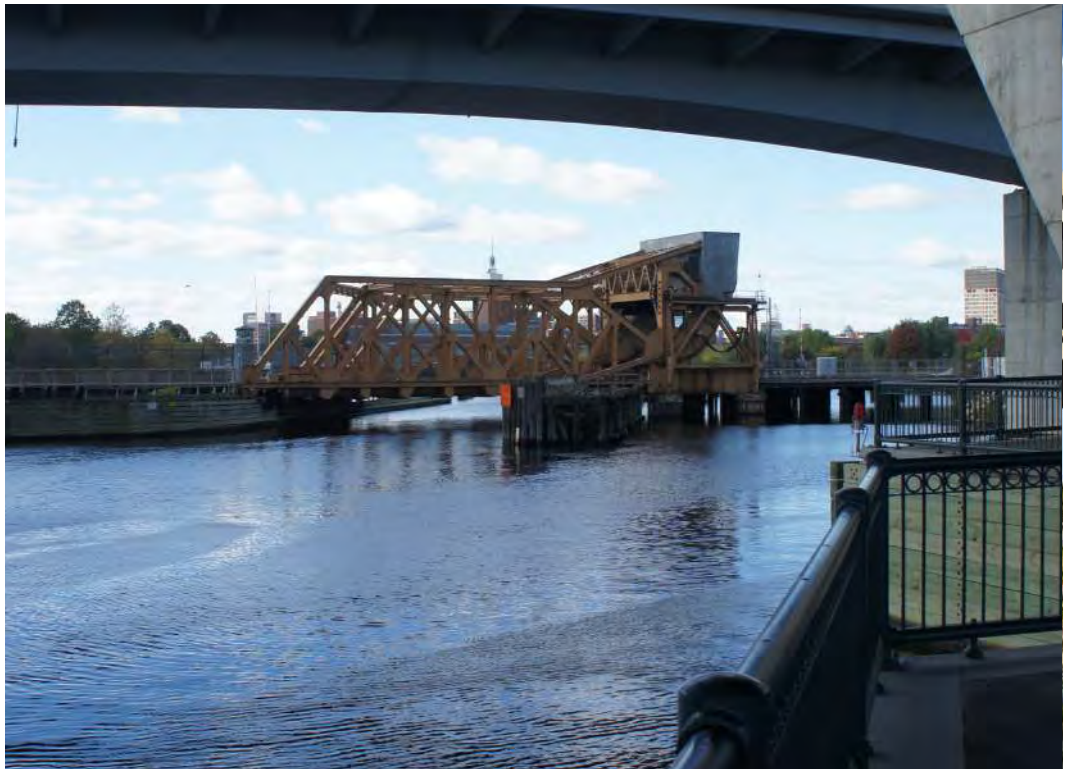
Photo 2 View of Draw One Bridge underneath Zakim Bridge, looking west from Cambridge.
