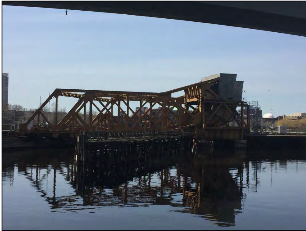
Figure 10. Draw 1 Bridges, looking west.
