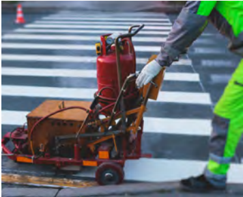
Refreshing crosswalks and pavement markings
