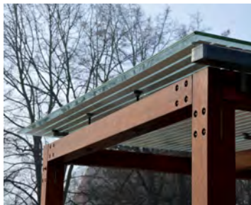
Installing bus-shelter green roofs
