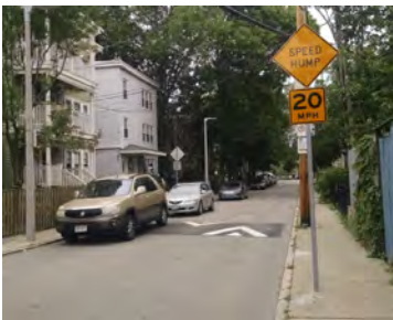
Installing speed humps on neighborhood streets
