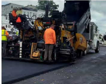
Repaving damaged sections of roadway
