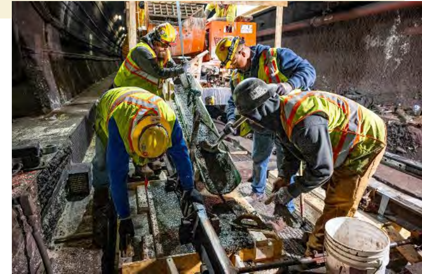
Repairing concrete slabs
