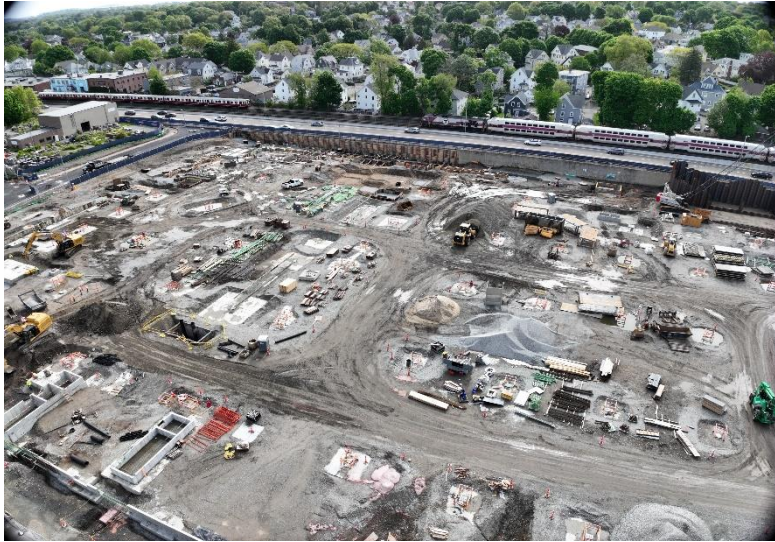
New Quincy Bus Maintenance Facility
