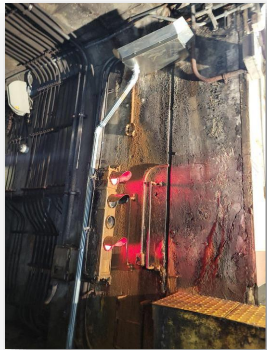
Sheet metal installed. New drain to prevent water leaking on the 10-5 signal, northbound pit just after the first car marker.
