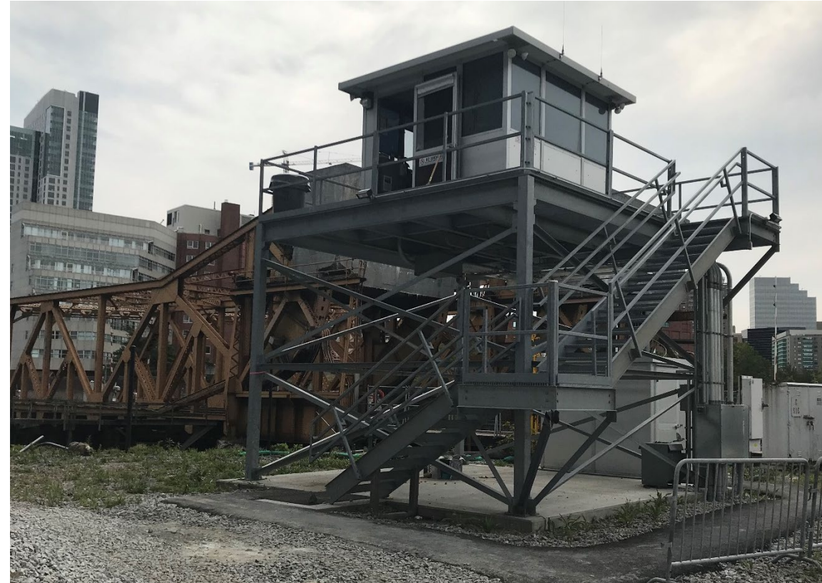
Current Control Tower A structure
