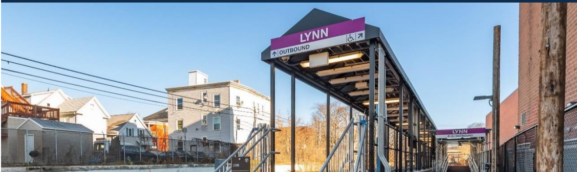
Commuter Rail temporary platform at Lynn to continue supporting service on the EJ Corridor.
