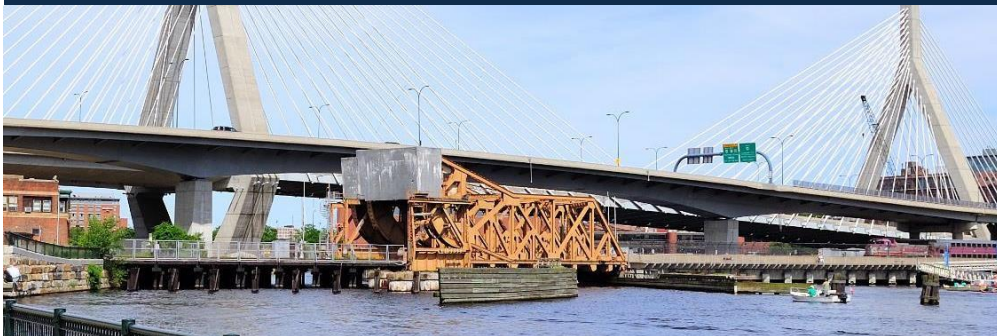
Existing 1930's North Station Draw 1 Bridge.
