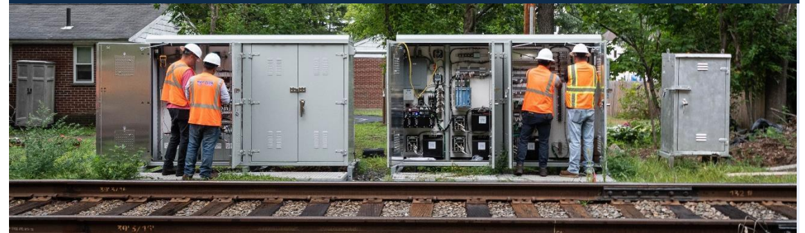
Maintenance-of-way crew performing work at our ROW.
