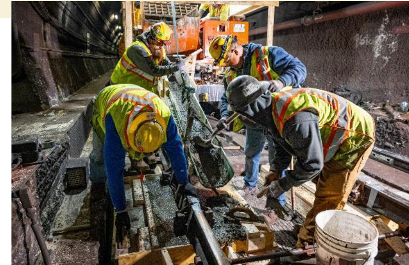
Repairing concrete slabs
