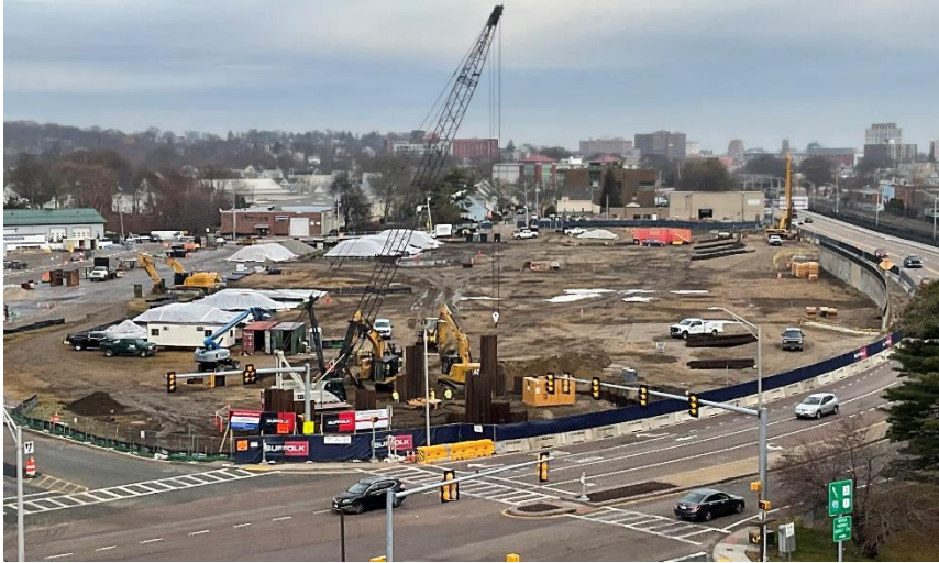
New Quincy Bus Maintenance Facility
