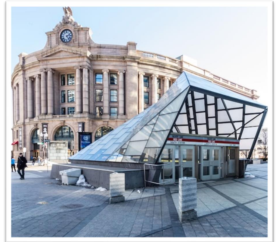
DPU Rail Transit Safety is located above the South Station rail terminal in downtown Boston.
