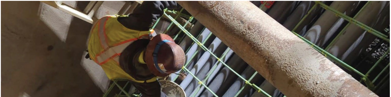
Construction continues on Codman Yard duct banks
