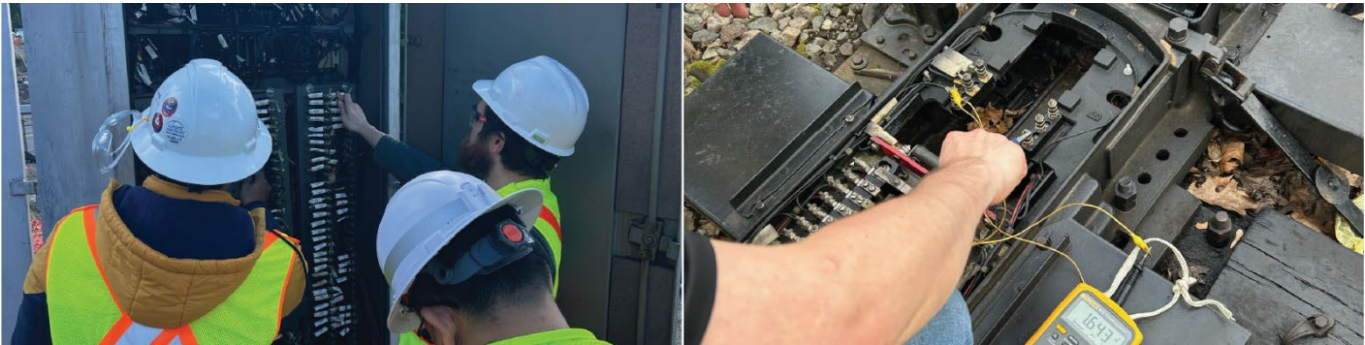
Signals work completed during the Ashmont Branch/Mattapan Line surge
