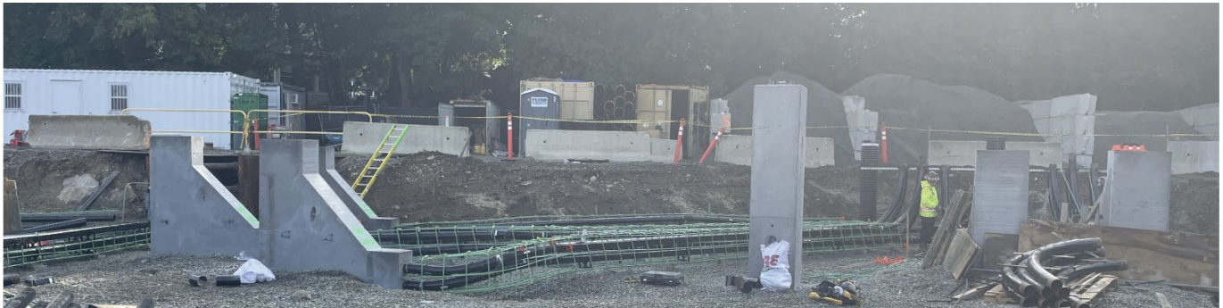
Construction of duct banks continues at Codman Yard
