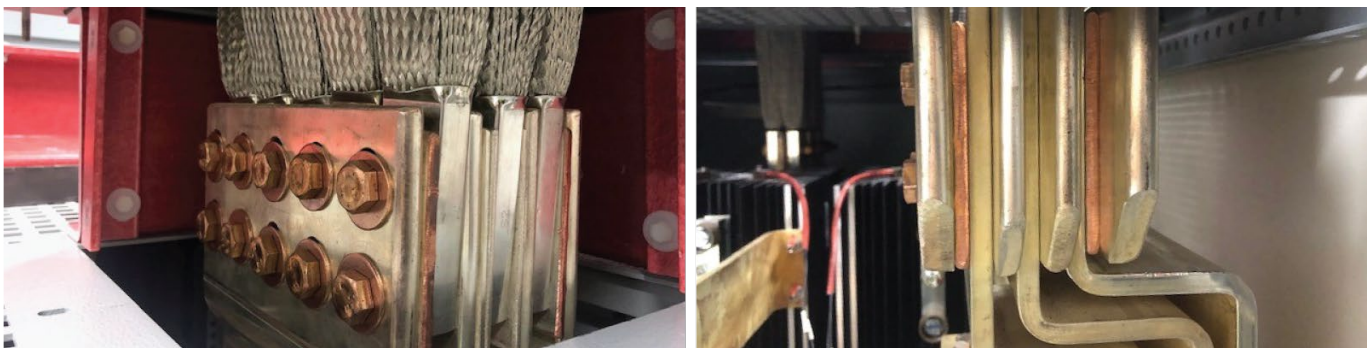
New electrical connections installed at Oak Grove
