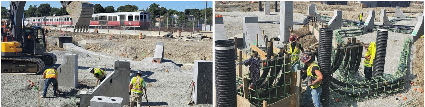
Duct bank construction in Codman Yard
