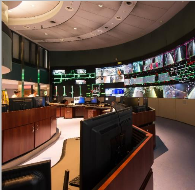
OCC ROW worker location pilot
