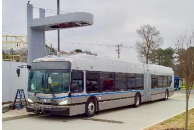
A Silver Line Battery Electric Bus (BEB) with an example of en-route charging equipment
