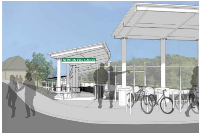
Rendering of the upgraded, fully accessible, Newton Highlands Station on the Green Line. Upgrades will include raised platforms, detectable warning strips, and two accessible routes to platforms as shown in the image
