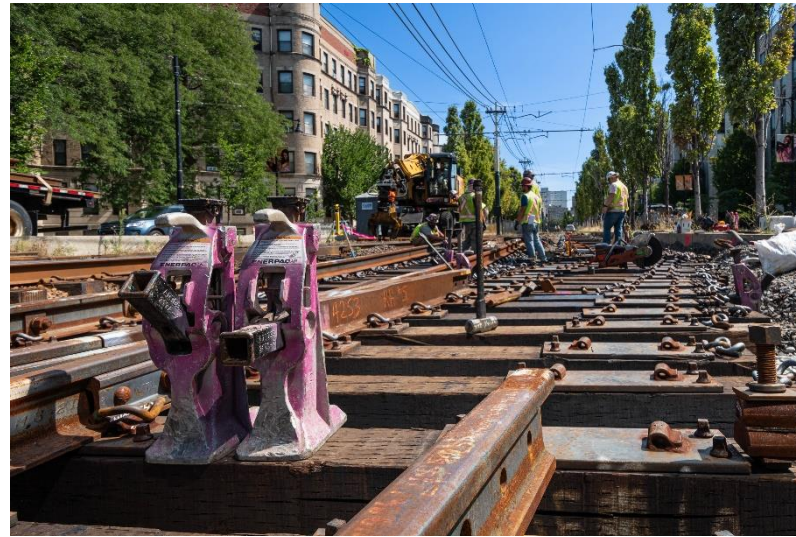
Track maintenance and replacement on the Green Line's E Branch
