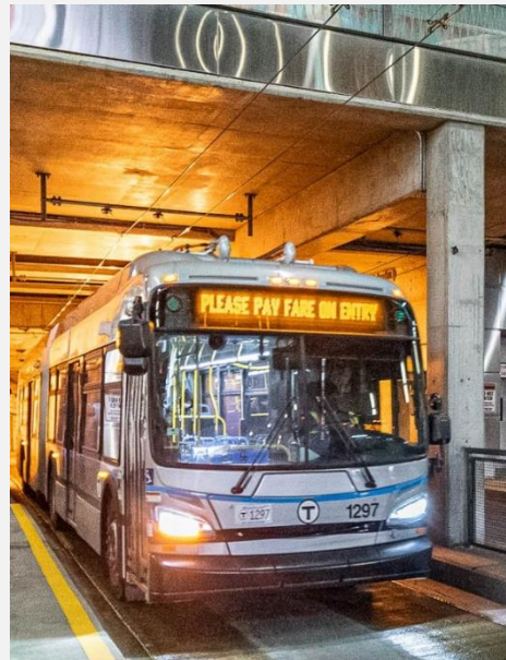
Silver Line's 60ft battery-electric bus with electric charging infrastructure
