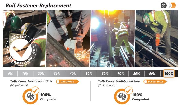
✓ This Week | Concrete repairs were completed this week and crews demobilized from the Tufts Curve area. This rail fastener replacement work was required by the FTA's Special Directive 22-4, and by completing these upgrades we have been able to remove a speed restriction that had been in place since 2019
