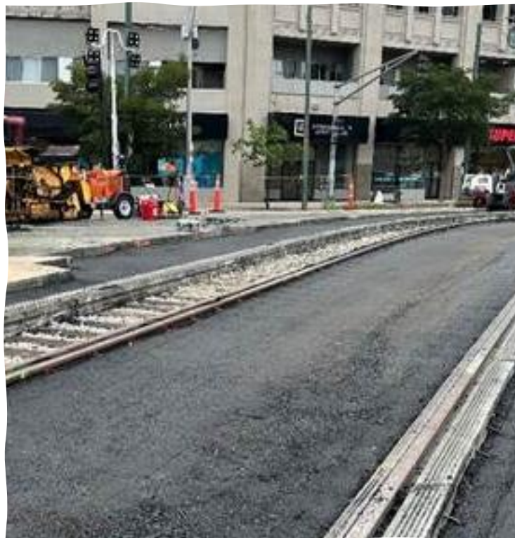
Paving at Packard's Corner
