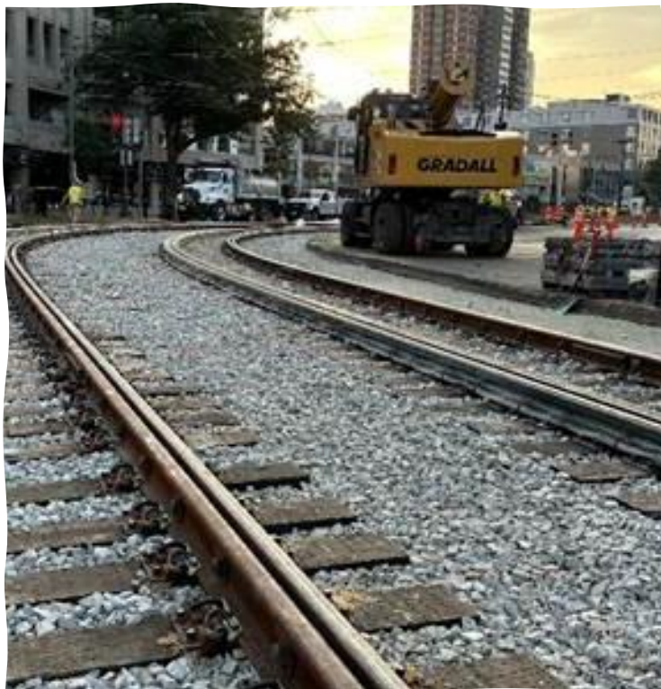
Completed new track at Packard's Corner
