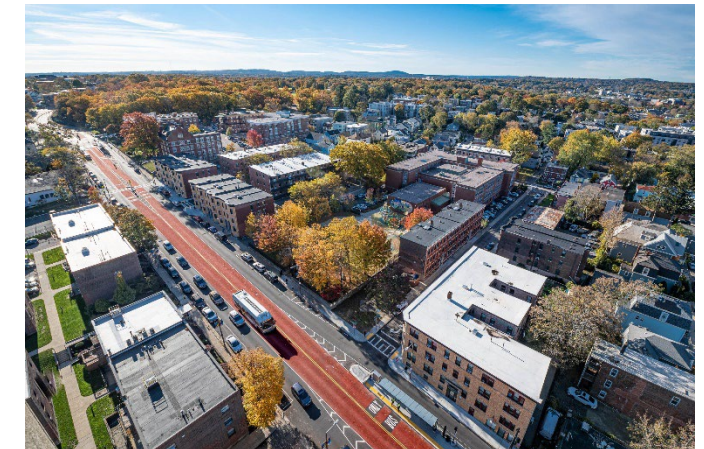
Aerial view of center-running bus lane and transit supportive infrastructure at Columbus Ave
