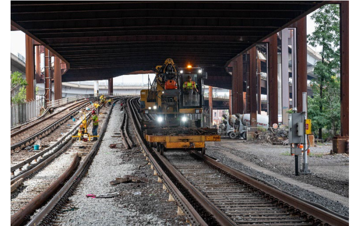
Track maintenance and replacement on the Orange Line
