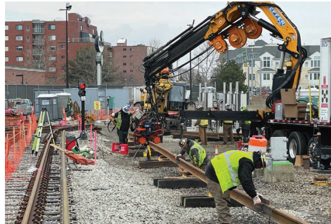
Installing new tracks at Wellington Yard
