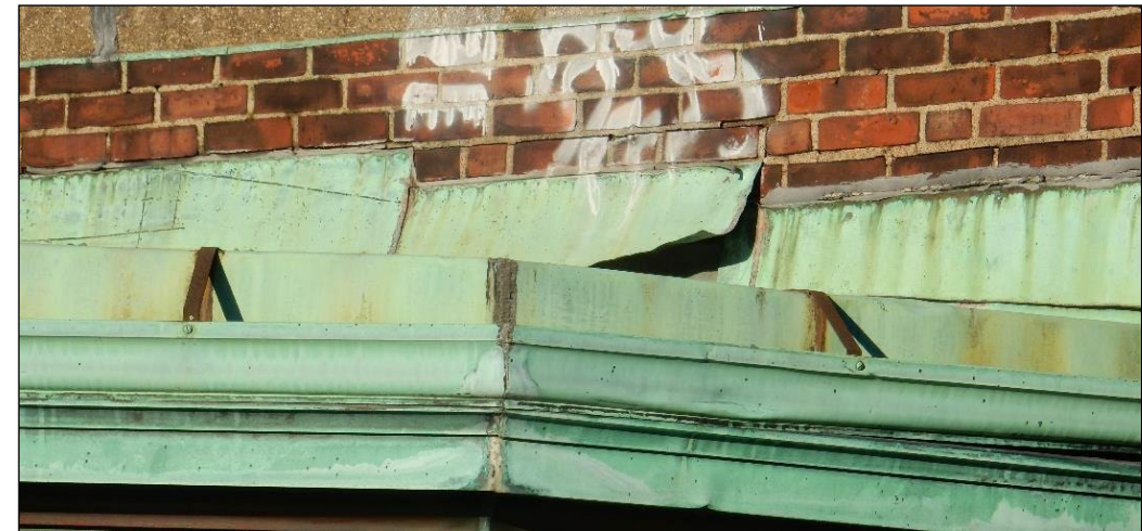
Bent and damaged copper flashing
