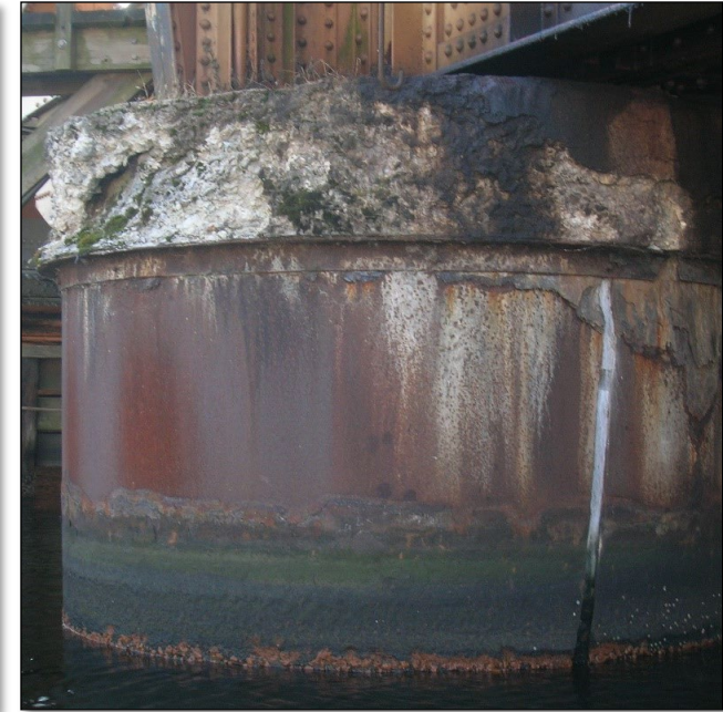
Picture of Bridge Caisson showing deterioration
