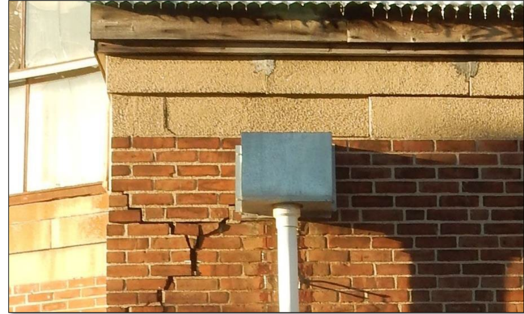
Severely cracked and displaced brickwork
