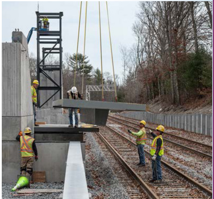
Platforms being installed at East Taunton Station, February 2023.
