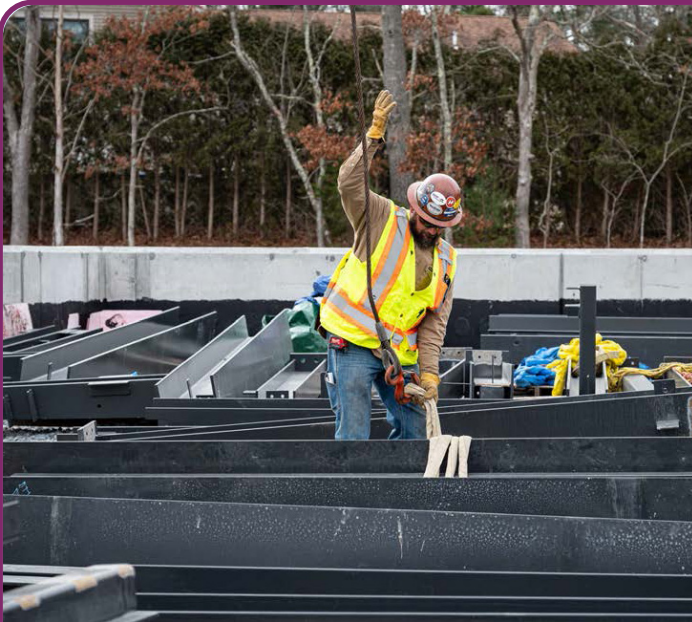
Platforms being installed at East Taunton Station, February 2023
