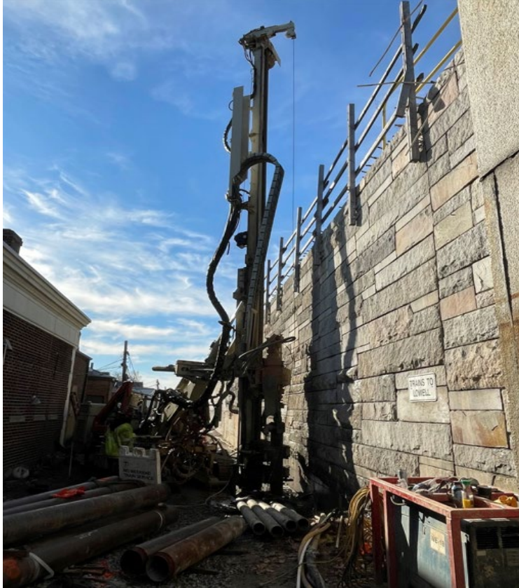
Micropile Work Behind Thompson Street (December 2022)
