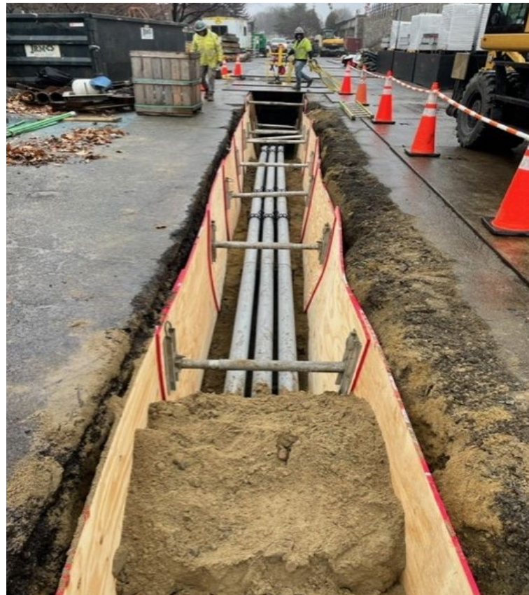
Backfilling of Eversource Ductbank at Laraway Road (January 2023)
