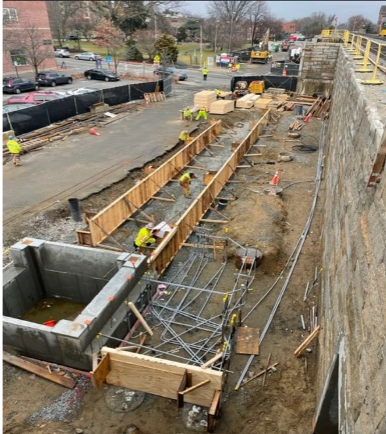
Form work for West Headhouse Grade Beams (January 2023)
