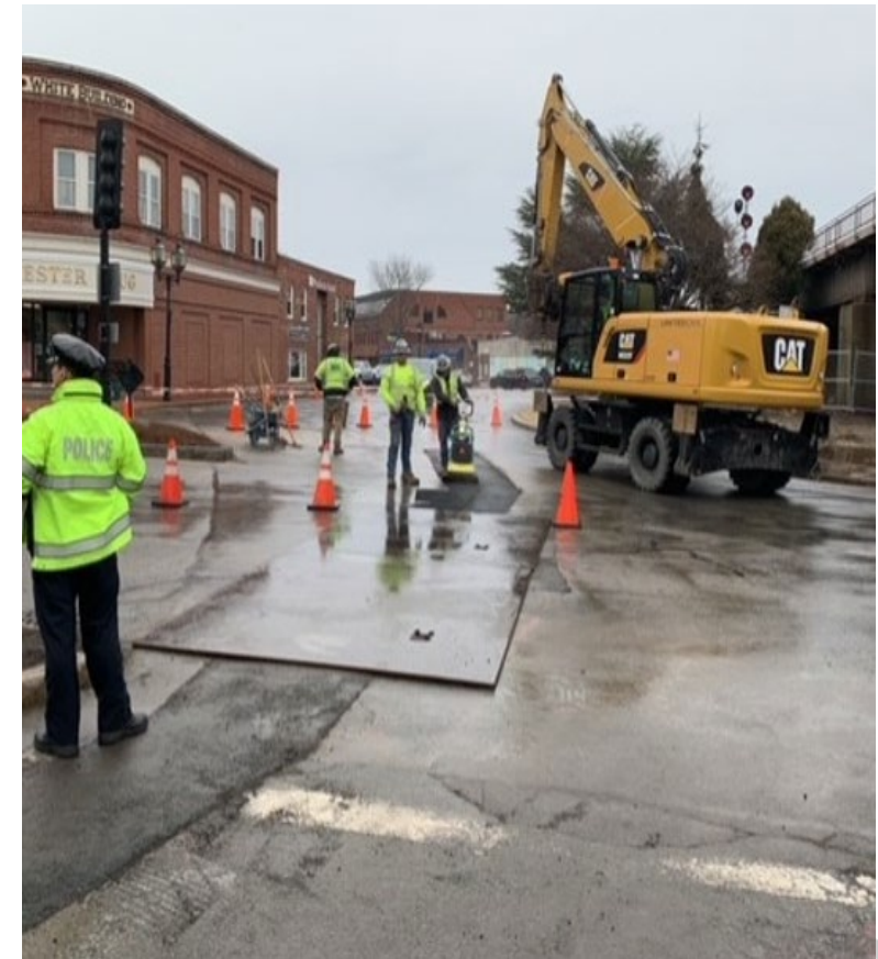
Eversource Work at Quill Rotary Installing Main Station Power (February 2023)
