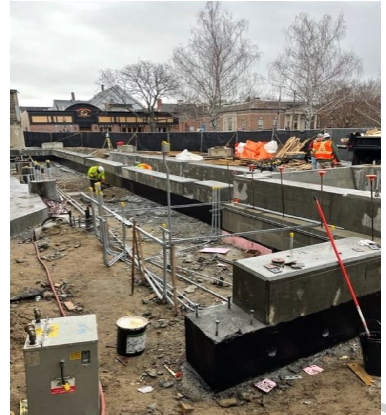
Waterproofing East Headhouse Grade Beams at the Aberjona Lot (January 2023)
