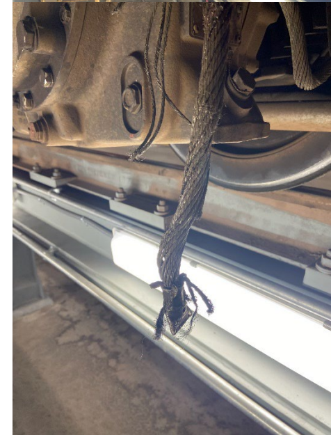
Broken Ground Strap
